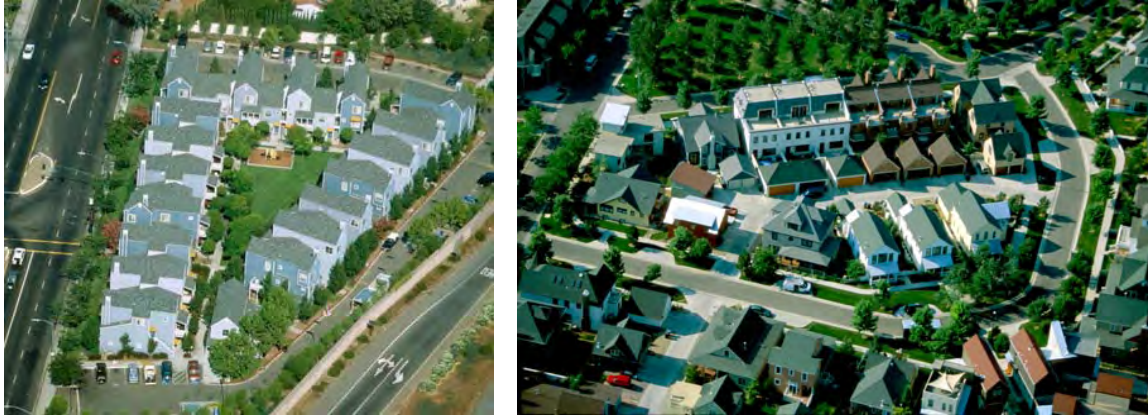
Figure 3-27-B: Mixed-density residential at approximately 12 dwelling units/acre
