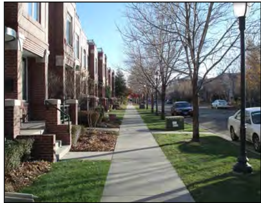
Fig. 3-27-1: Ground-floor unit entrances
