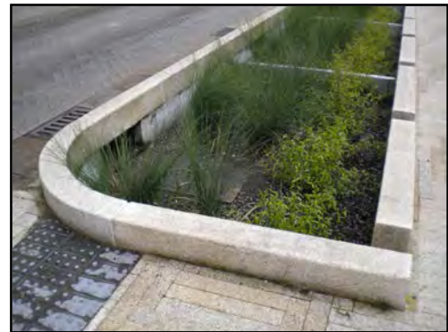
Fig. 3-27-BB: LID stormwater management feature
