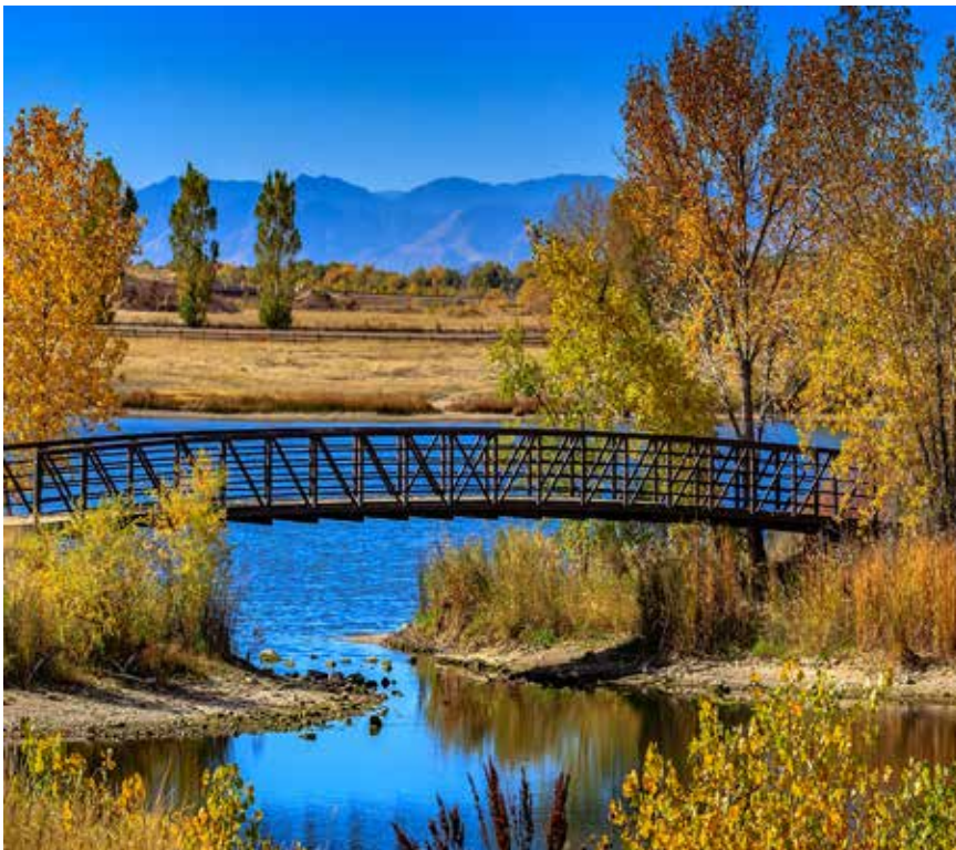
Riverdale Regional Park Bridge
