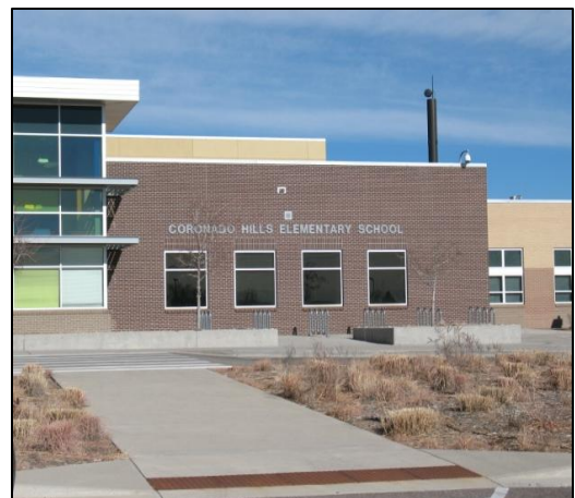
Coronado Hills Elementary School north of Coronado Parkway at E. 83rd Place.
