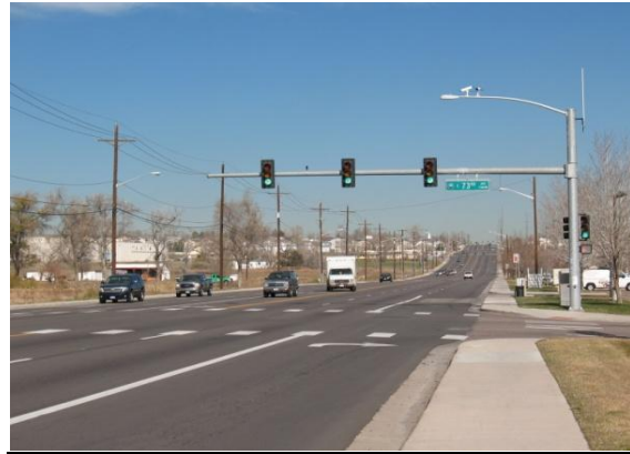
A major arterial in Welby, Washington Street provides essential north/south connections on the west side of Welby.
