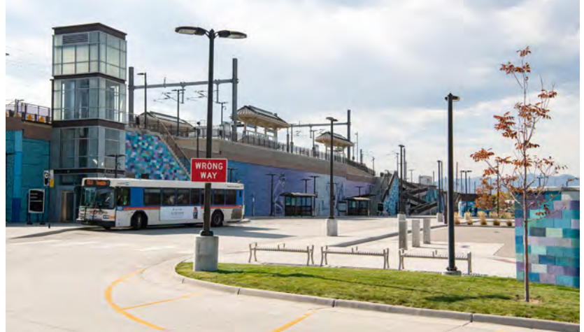
Figure 17: RTD G Line Clear Creek Station at Federal Boulevard
