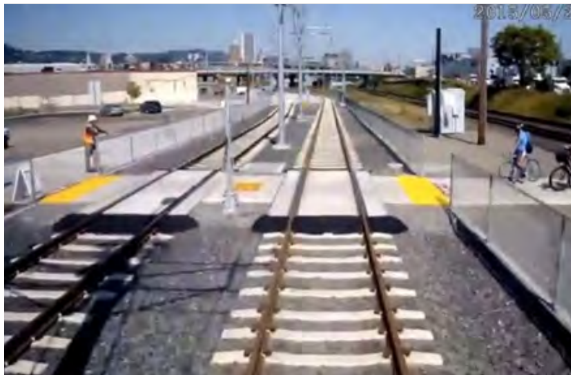
Figure 57: Sample At-Grade Rail Crossing Treatments (Source: Trimet)
