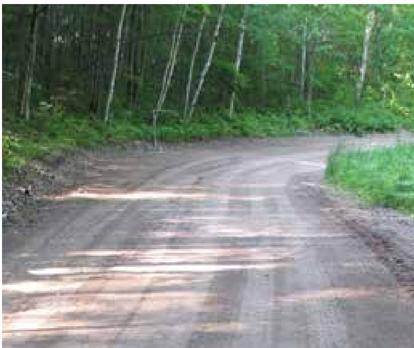
Figure 3.18: Curved Gravel Road (source: EMTSP)
