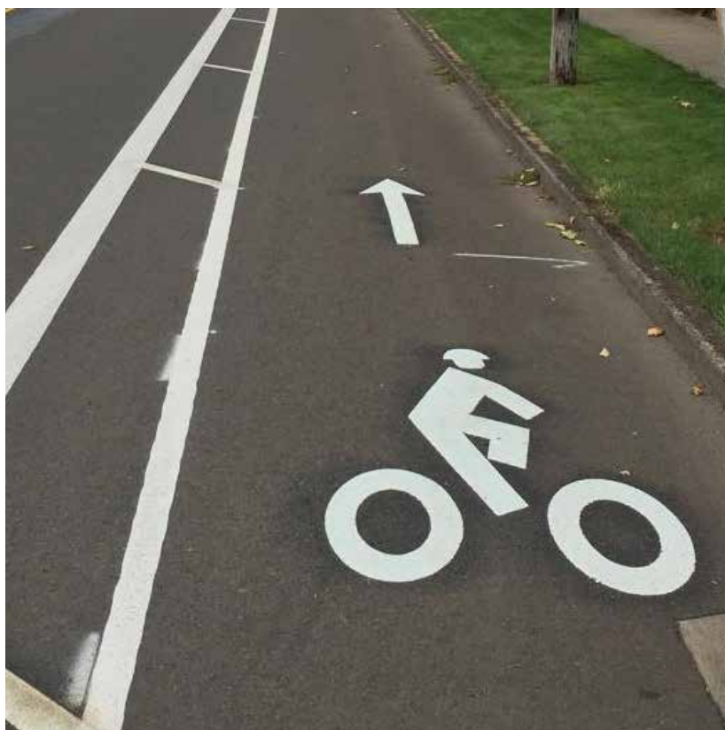
Figure 5.4: Buffered Bicycle Lane
