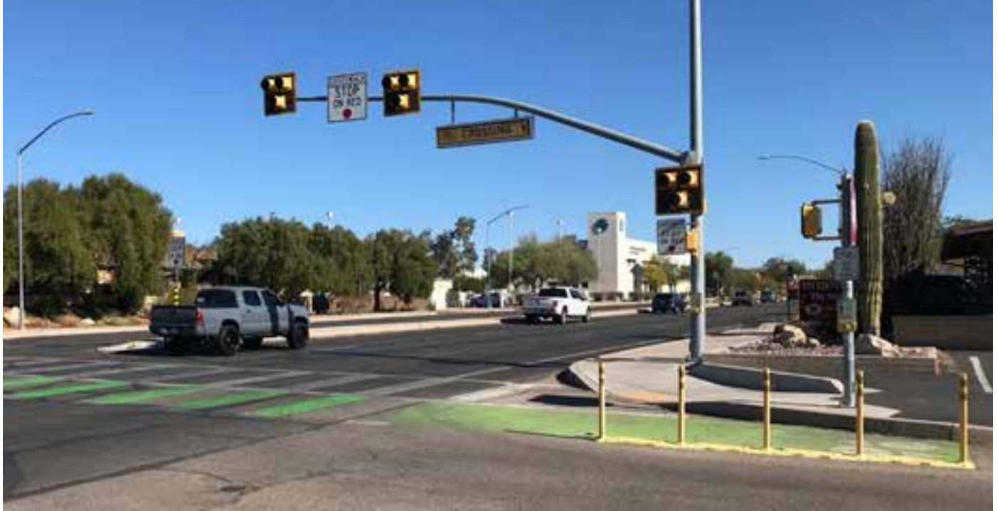
Figure 2.9: Example of an Enhanced Crossing Treatment with Dedicated Bicycle Striping and Signals (source: Fehr & Peers)
