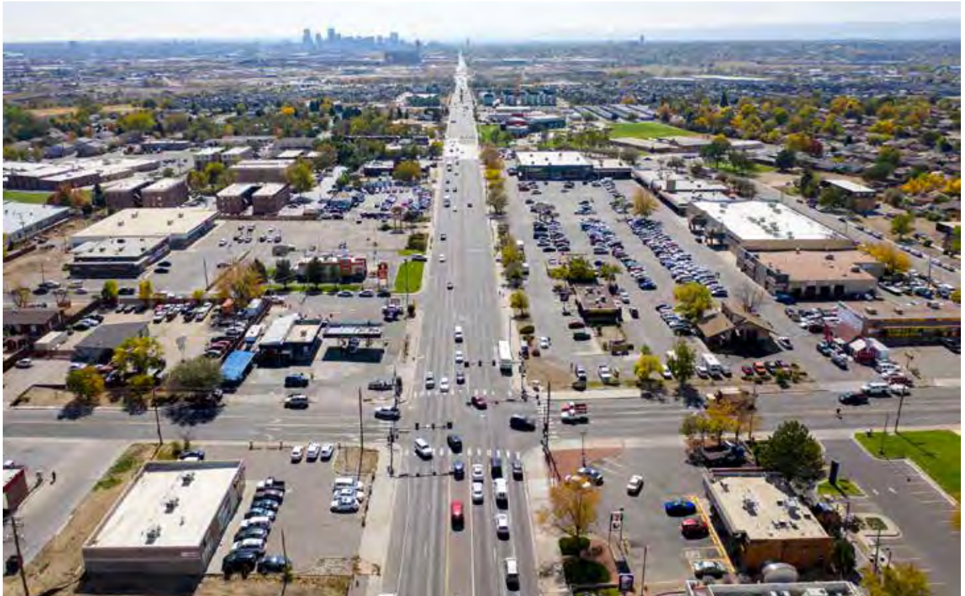
Figure 3.1: Aerial of Intersecting Roadways in Adams County (source: Design Workshop)
