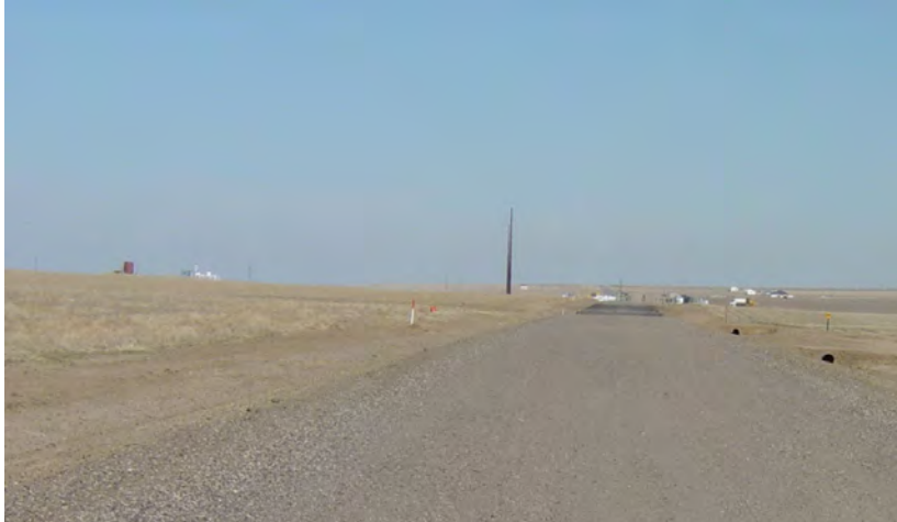
Figure 24: Unpaved Section of Imboden Road
