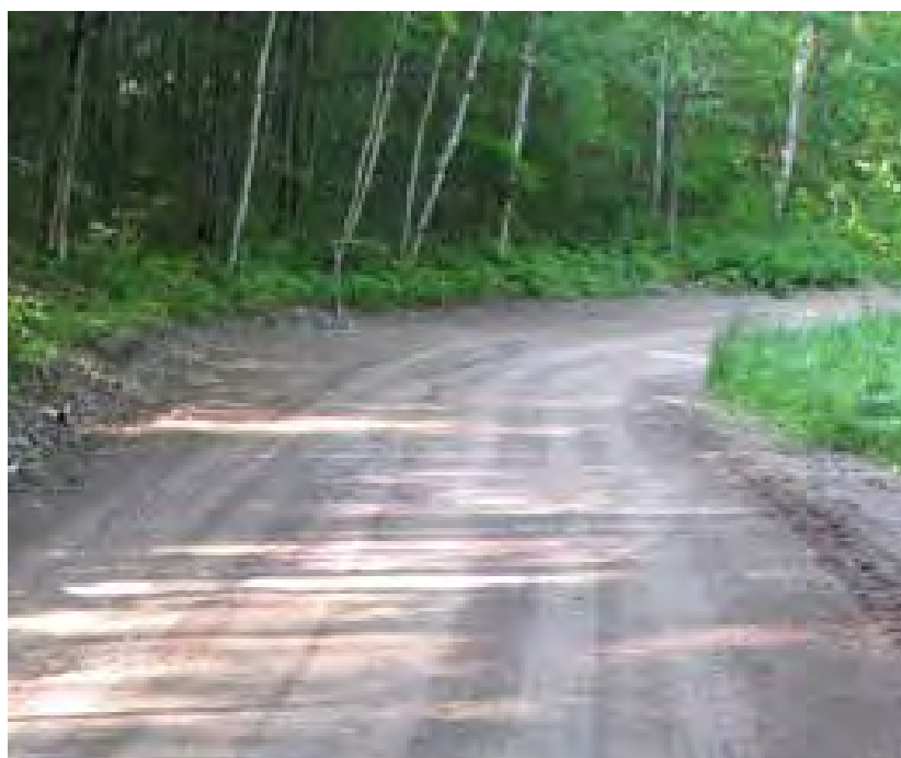
Figure 3.18: Curved Gravel Road (source: EMTSP)
