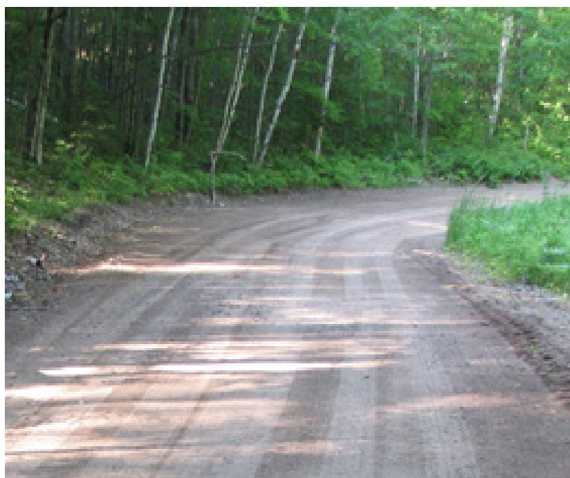
Figure 3.18: Curved Gravel Road (source: EMTSP)
