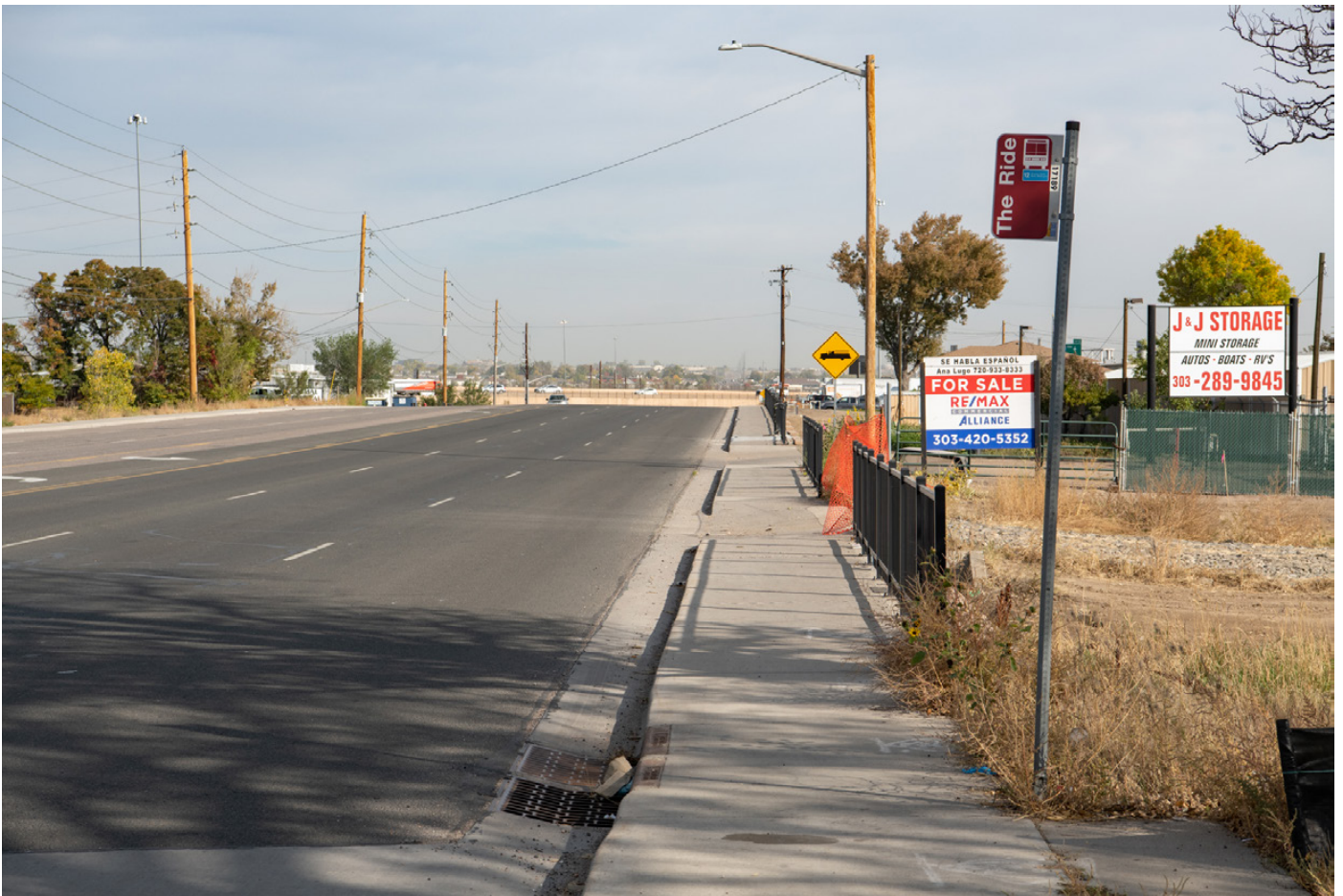
Figure 2.19: Sidewalk and RTD Bus Stop on Washington Street (source: Design Workshop)
