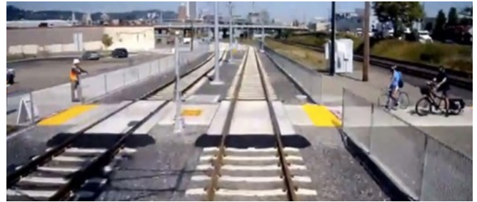
Figure 2.22: Sample At-Grade Rail Crossing Treatments (source: Trimet)
