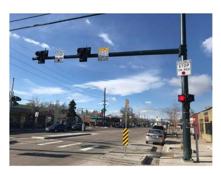
In addition to near-term opportunities adjacent to the commuter rail station, pedestrian connections all along the corridor could be improved through implementation of enhanced crossings. This can be accomplished through installation of treatments like High Intensity Activated Crosswalk (HAWK) signals (Figure 2.8), which serve as a stop control for traffic while pedestrians cross. These can be paired with green-backed intersection markings for bicyclists like the example shown in Figure 2.9.
