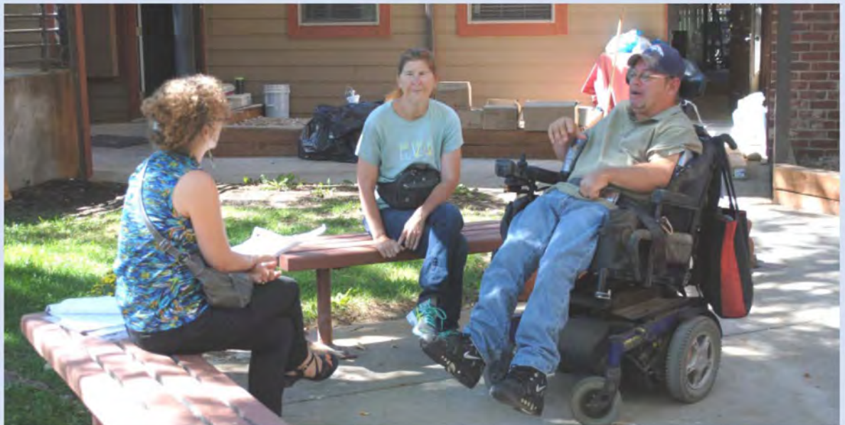
Renovated Sage Court apartments by Thistle Communities provide safe affordable homes for persons with disabilities in Boulder, Colorado.
