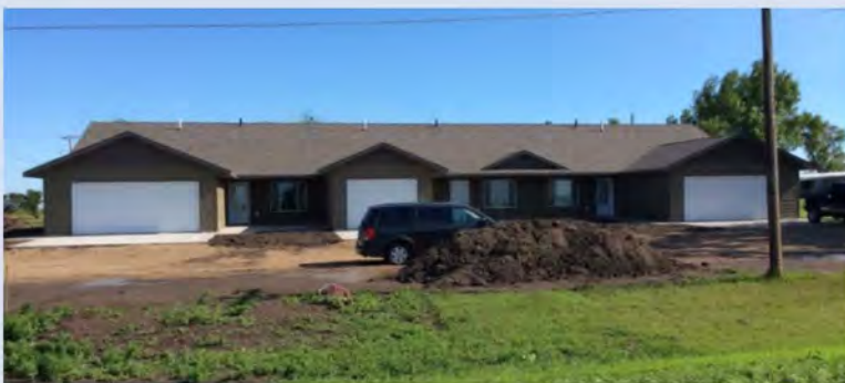
The Doland Tri-Plex emerged to sustain affordable housing for residents in Doland, South Dakota.
