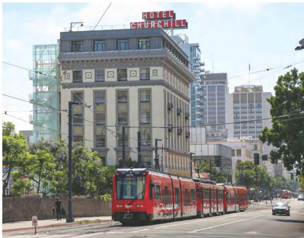
The Churchill Renovation. Occupancy expected to begin summer of 2016. Photo credit: San Diego Housing Commission
