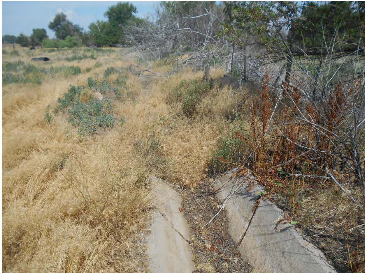
Photo 2: View to the east of TM-A9-Swale-01, located on the northern side of wetland TM-A06-WT-01. Stream TM-A08-STR-01 can be seen in the lower half of this photograph as a cement lined irrigation ditch. No OHWM, defined bed, defined banks, or scour were observed within TM-A09-Swale-01; the swale is not likely a jurisdictional WOTUS.
