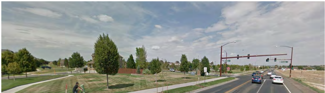
New Retail, Residential, and Open Space Development on 128 th and Oneida Street.
