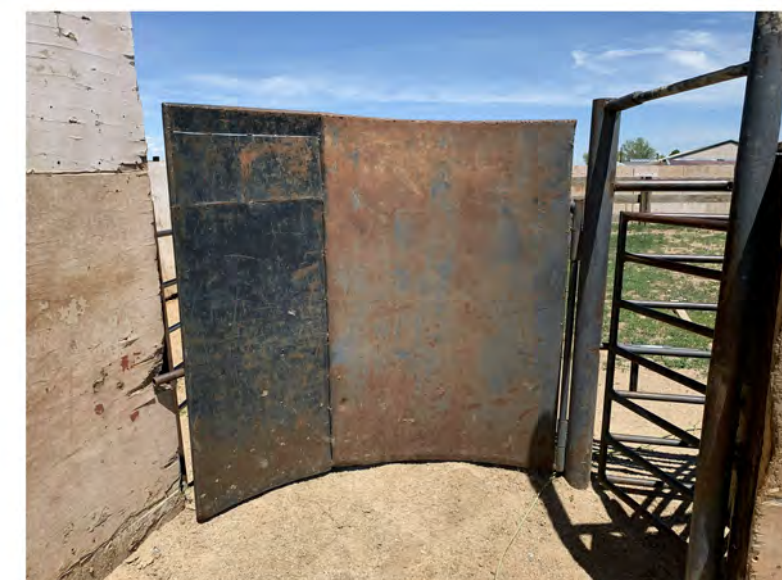
(8) NORTH WEST STEEL GATE
