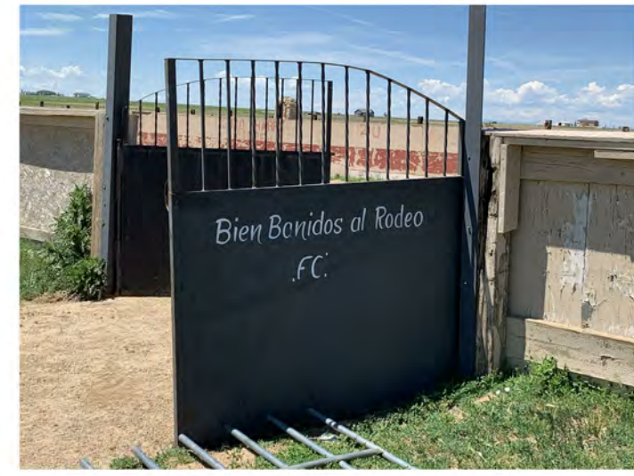
(1) MAIN STEEL GATE
