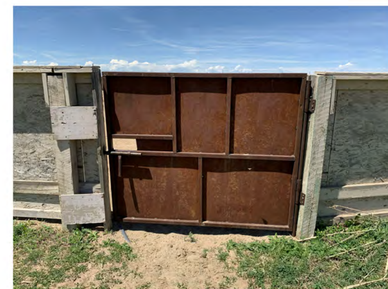
(4) SOUTH EAST STEEL GATE
