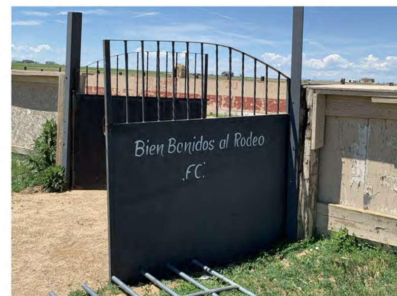
(1) MAIN STEEL GATE
