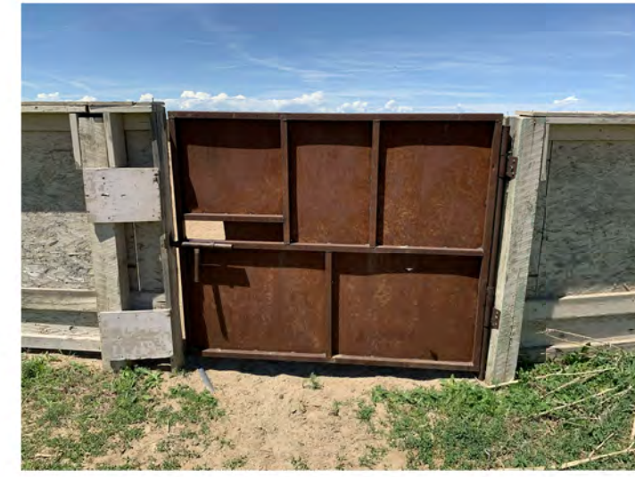
(4) SOUTH EAST STEEL GATE
