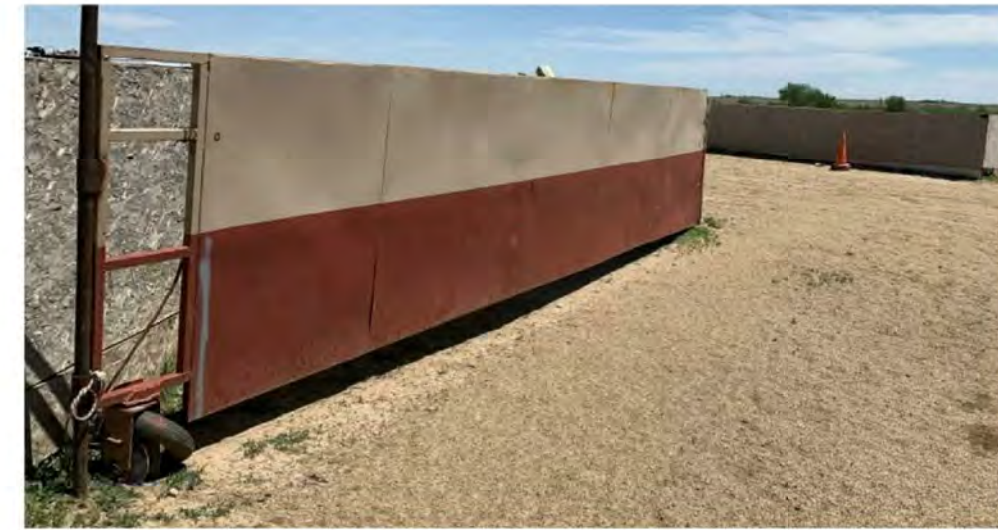
(7) SOUTH WEST STEEL GATE
