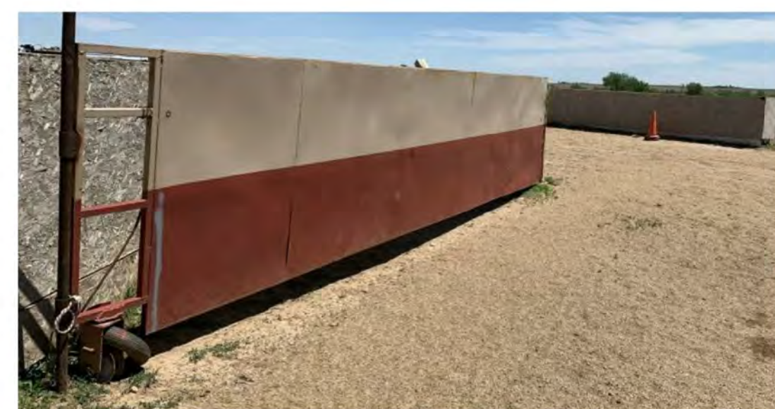
(7) SOUTH WEST STEEL GATE
