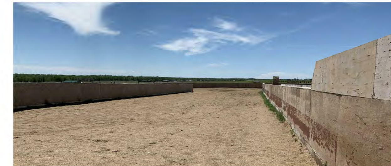
(12) INTERIOR VIEW LOOKING SOUTH
