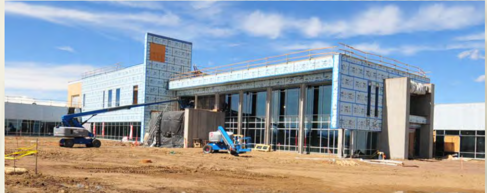
Front Lobby Construction – April 2017
