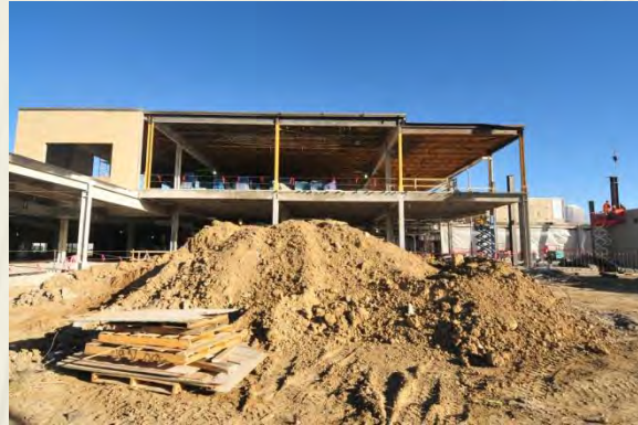
Main Entrance – October 2016
