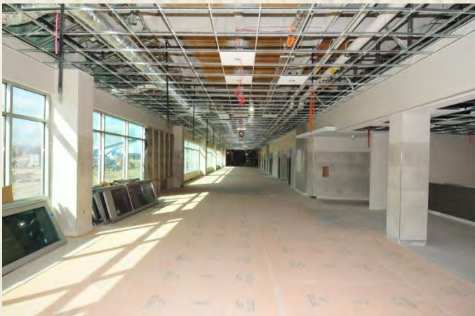
Main Lobby – March 2017
