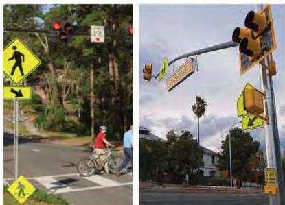
SAFE PLACES TO CROSS - High-Intensity Activated Walk ("HAWK") traffic signals stop traffic when pedestrians need to cross
