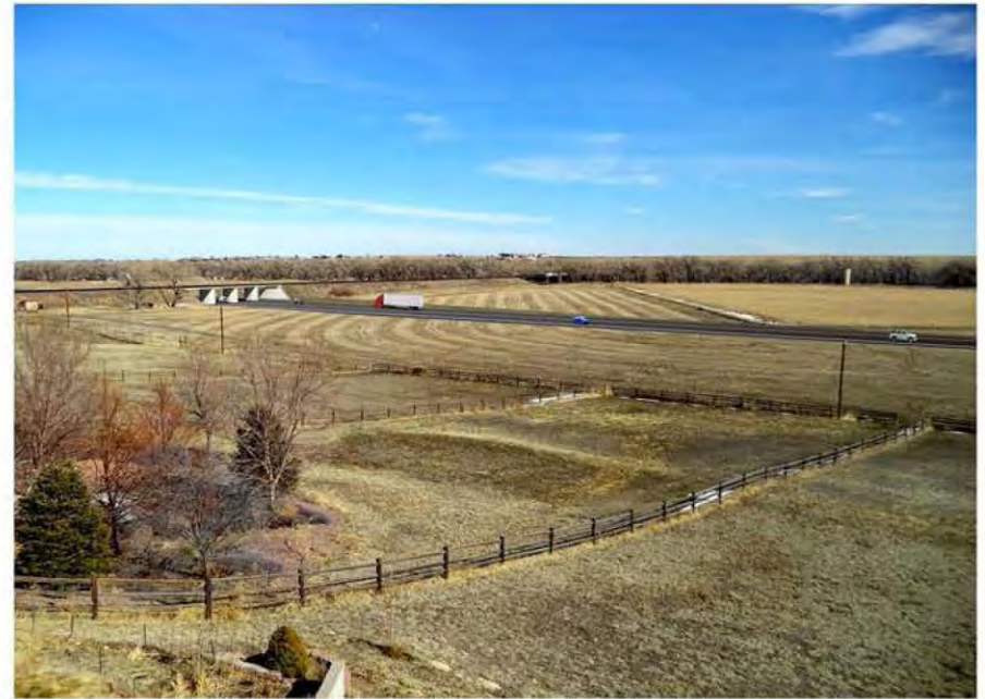
Railroad Crossing Underpass
