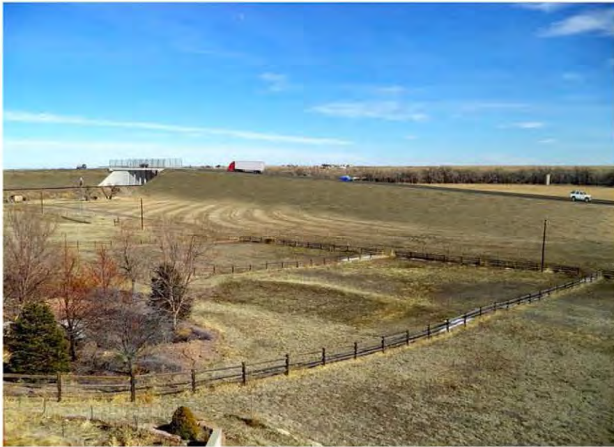
Railroad Crossing Overpass
