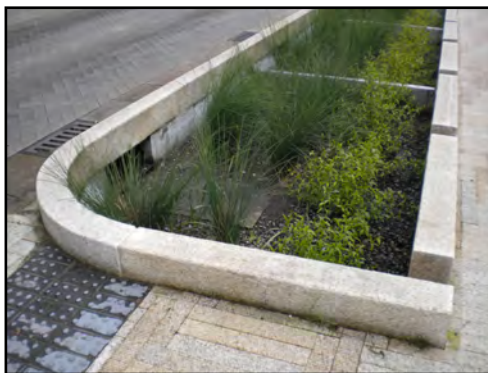
Fig. 3-26-BB: LID stormwater management feature
