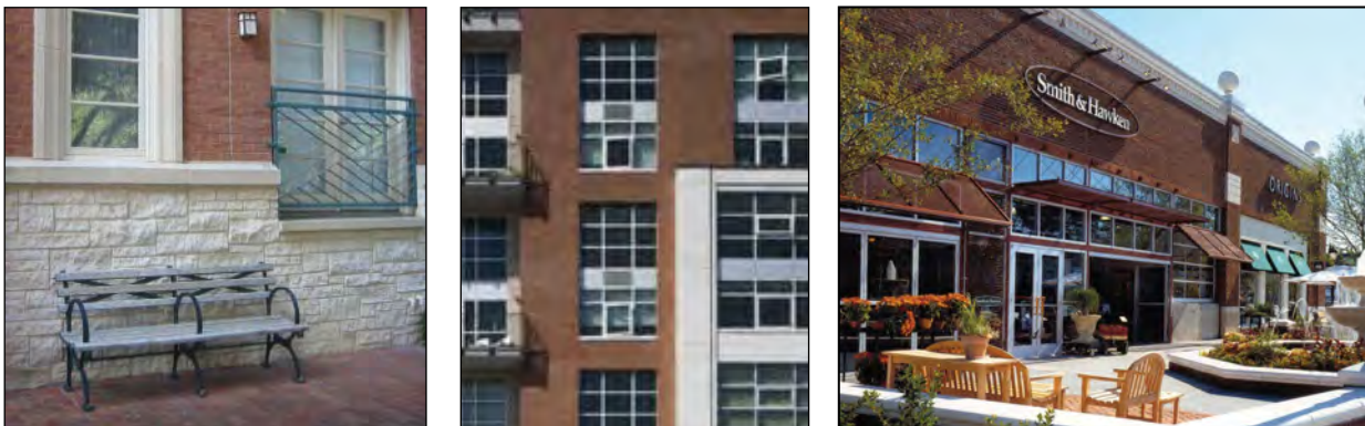
Fig. 3-26-W: Mix of building materials
