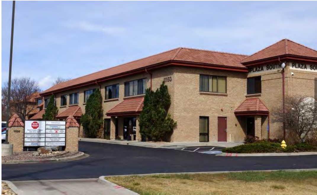
RENT 1 - 11150 Huron St, Building II
