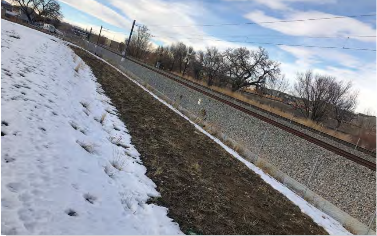
Photo 1 - Overview of light rail tracks and stormwater conveyance channel east of the project area. View is to the northwest.
