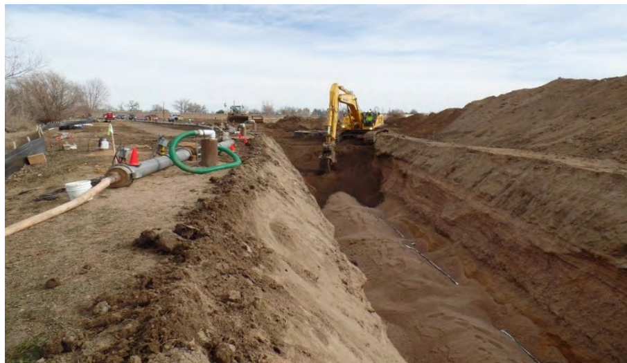
Figure 10-9: Examples of Open-Cut Construction Methods
