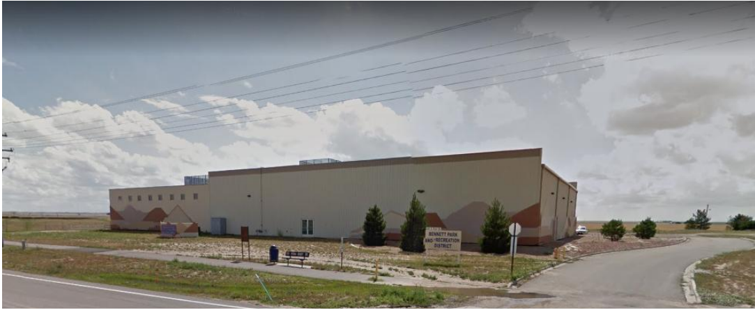
Bennett Parks and Recreation Facility, 455 S 1st St, Bennett, CO 80102.
