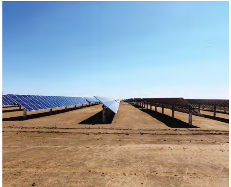
Similar solar panels at nearby Victory Solar Project. The maximum height of the panels is approximately 8 feet.
