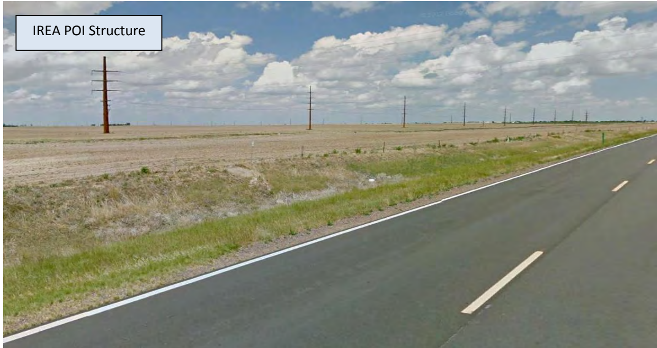
Figure 2 IREA/Pioneer POI & Transmission Line: Approaching from West & East Colfax
