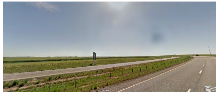
View of SD Interceptor alignment area from E-470 looking east. Views of roadway and open grasslands, with views of DIA in the distance.
