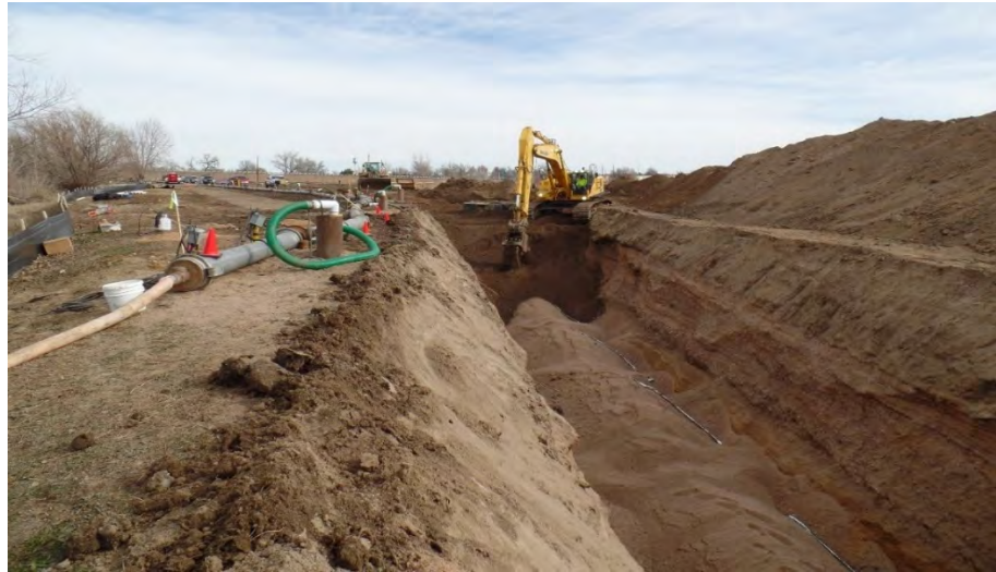
Figure 10-9: Examples of Open-Cut Construction Methods
