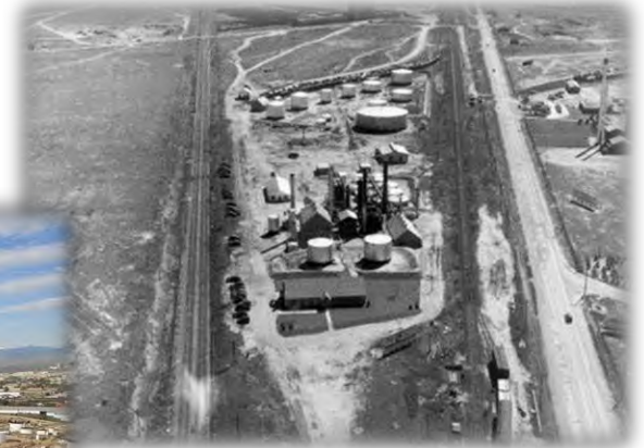
Plant 2, originally built in 1937
