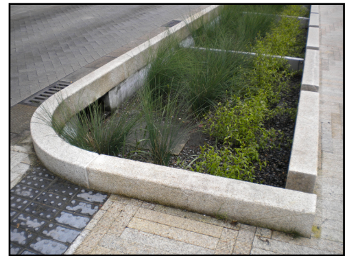
Fig. 3-276-BB: LID stormwater management feature
