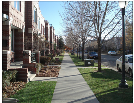
Fig. 3-276-I: Ground-floor unit entrances
