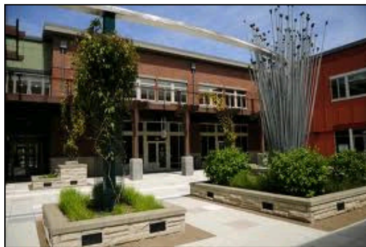
Fig. 3-276-P: Buildings arranged to create pedestrian-friendly spaces
