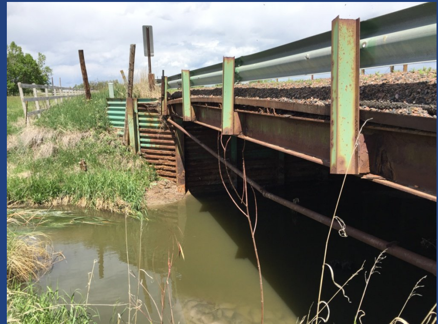
West edge of bridge looking north
