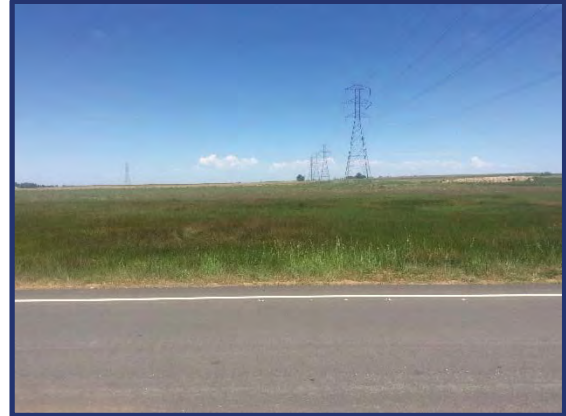
Image #8 – County Rd. 2 Crossing (Looking South)
