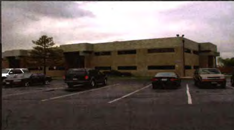
Honnen Building - Built in 1976
