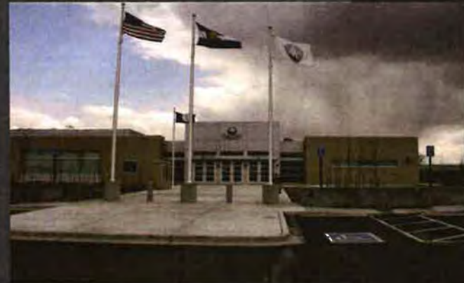
Sheriff HQ / Coroner Bldg Completed 2006
