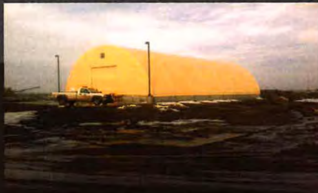
Strasburg Sand/Salt Building Completed 2015
