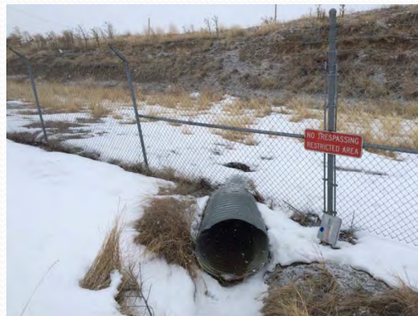
30" Storm Drain Outlet
