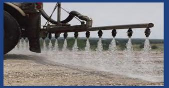
Rehabilitated roads require minimal maintenance for 3-5 years, at which time application of thin layer of polymer will continue to extend roadway lifecycle
