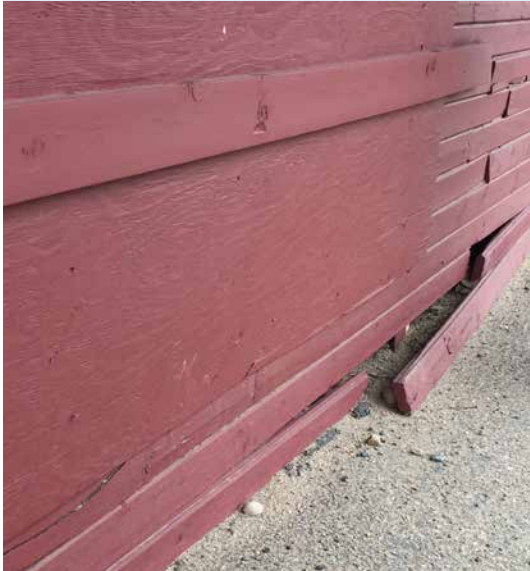
THE TONGUE AND GROOVE WOOD SIDING IS DETERIORATING
