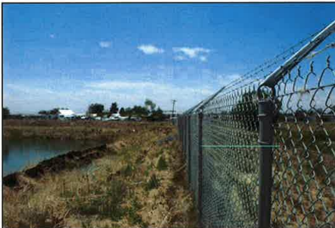
Figure 3 looking west at the failure surface
