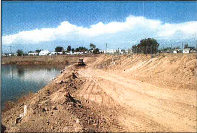
Figure 1 Location where inert fill was utilized to repair the embankment, looking NNW
