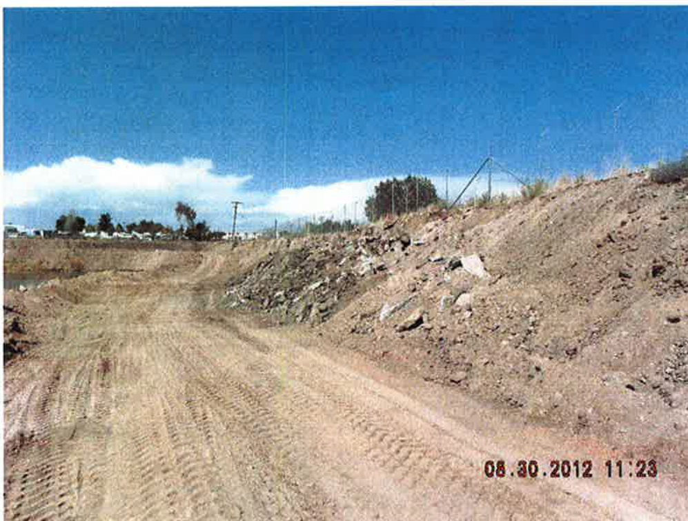
Figure 3 - Road constructed along north edge of pit
