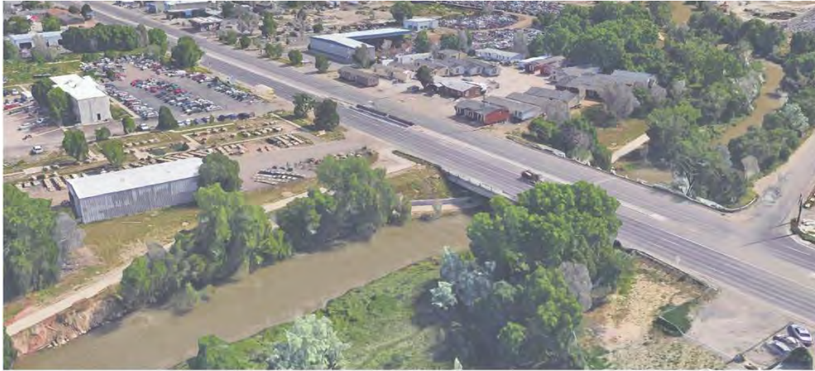
Sheridan Connection: The current conditions of the Federal Boulevard bridge over Clear Creek. The creek path will provide an important connection to Federal Boulevard from the Sheridan FasTrack Station. Current conditions however, do not encourage much pedestrian or biking activity.
