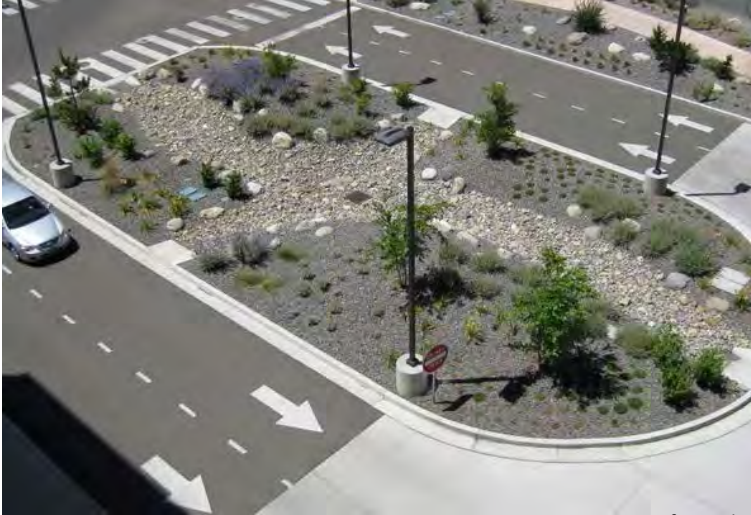
Photo 4-3: Rock-Lined Swale with Curb Cuts
