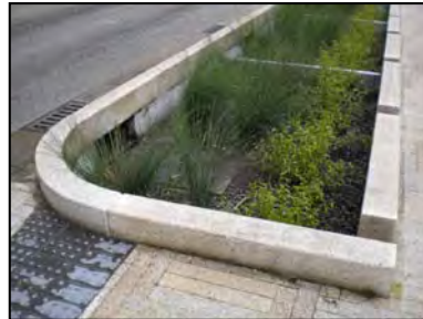
Fig. 3-26-BB: LID stormwater management feature
