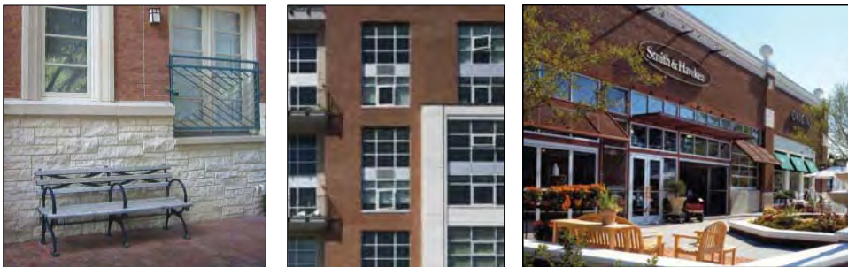
Fig. 3-26-W: Mix of building materials
