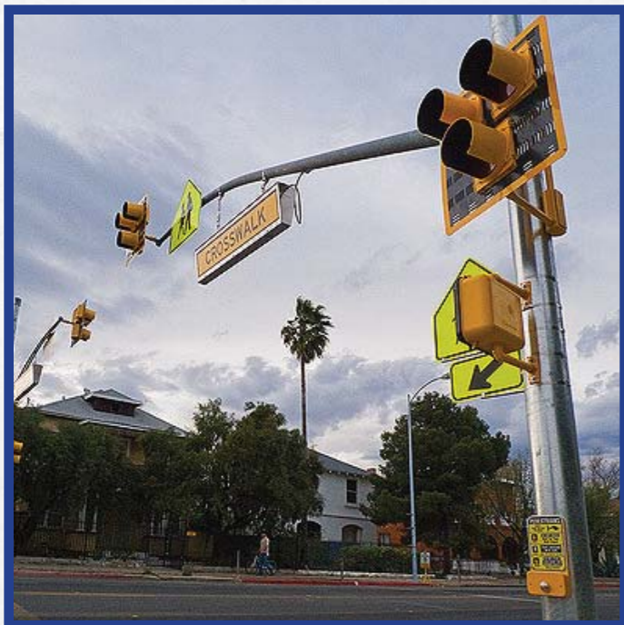
HUMAN-ACTIVATED SIGNALIZED CROSSWALKS ("HAWK" CROSSINGS)
