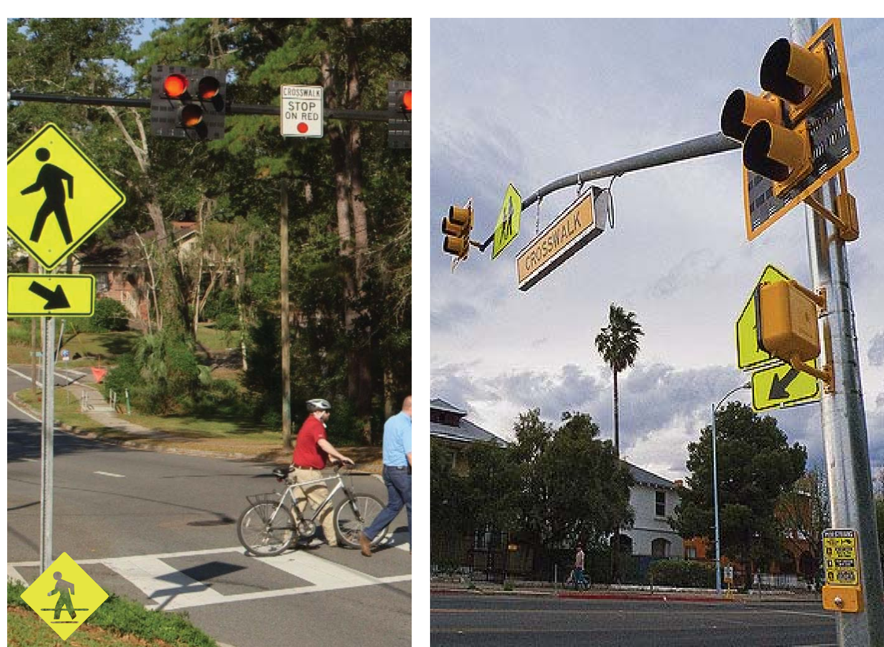
SAFE PLACES TO CROSS - High-Intensity Activated Walk ("HAWK") traffic signals stop traffic when pedestrians need to cross
