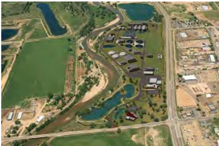
MWRD Northern Treatment Plant
