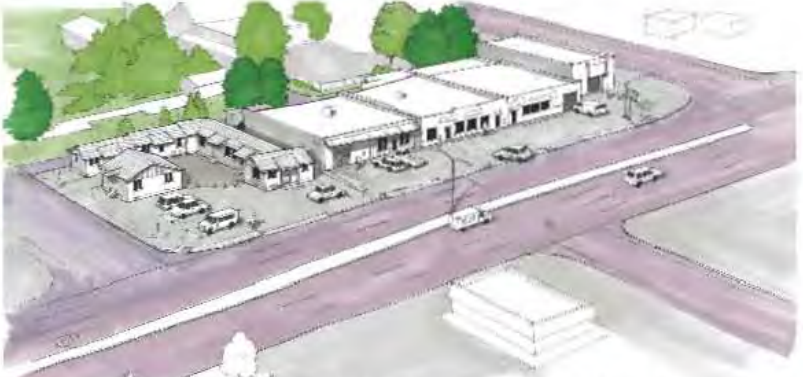
Current conditions (shown is the block between W.65th Avenue and W. Hawthorne Place): Extensive curbs, head-in parking, limited landscaping, lack of street trees do not provide a pedestrian friendly environment.
