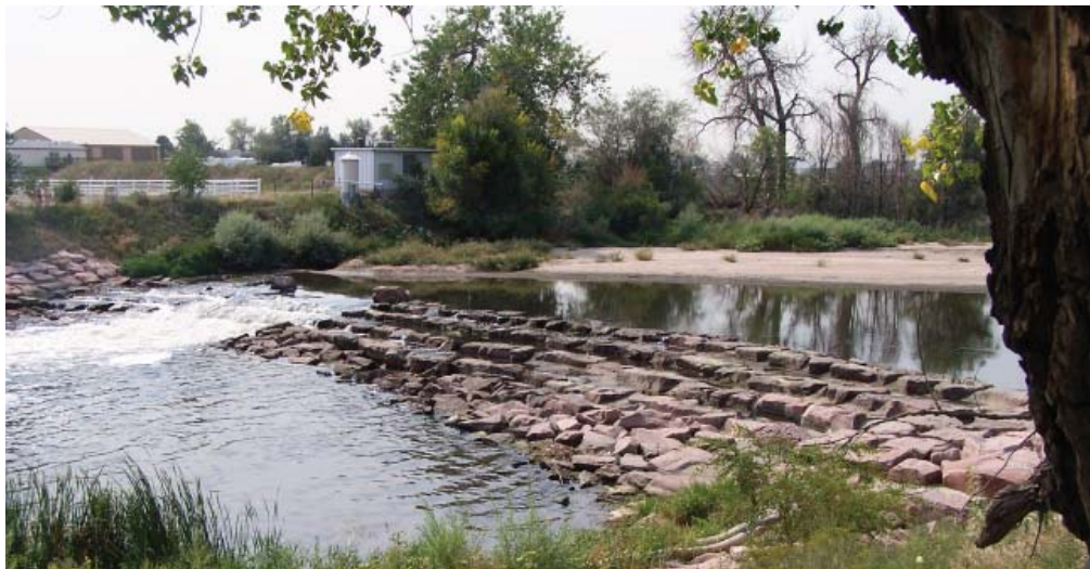
Drop structures designed to improve the water quality of the South Platte River were constructed at the eastern edge of the project area, adjacent to Adams County Regional Park.
