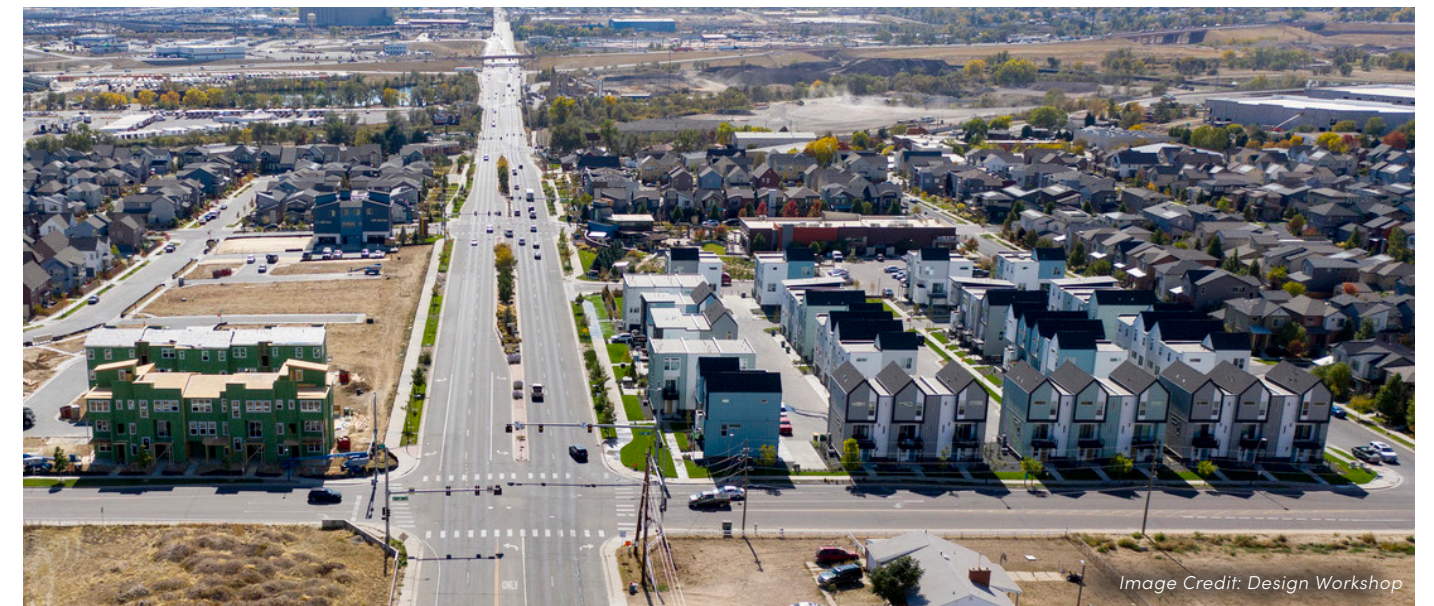
Figure 64: Pecos Street Between US-36 and 70th Ave
