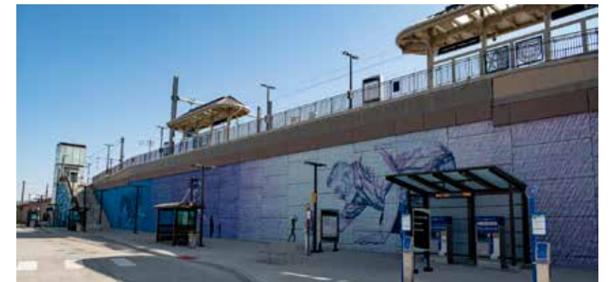
Figure 8: RTD Station on Federal Boulevard
