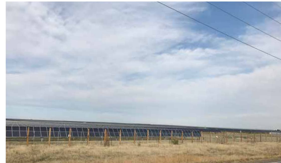
Figure 20: Solar Farm in Unincorporated Adams County
