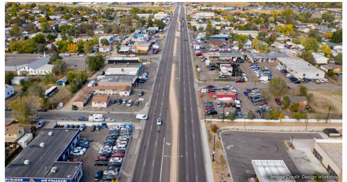
Figure 30: Aut-centric Commercial Activity North of West 64th Avenue on Federal Boulevard
