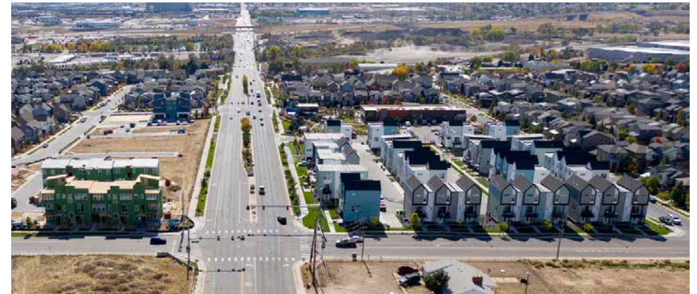
Figure 51: Pecos Street Between US-36 and 70th Ave
