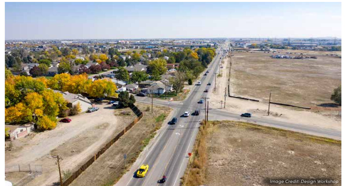
Figure 44: Brighton Road intersecting 104th Avenue
