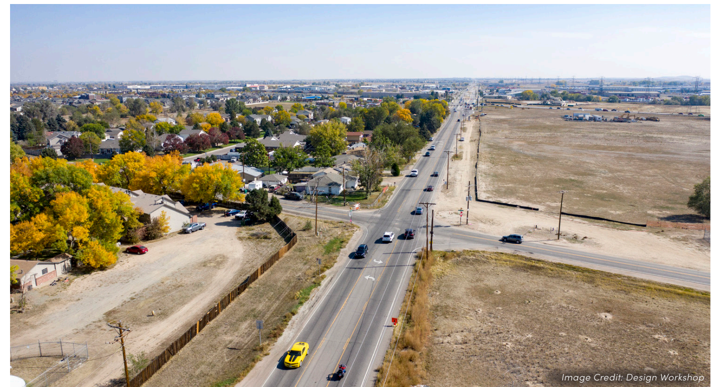
Figure 57: Brighton Road intersecting 104th Avenue
