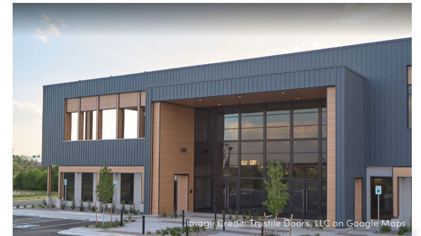
Figure 38: TruStile Doors New Facility
