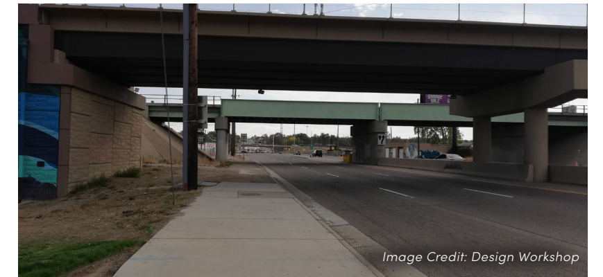
Figure 45: Federal and West 60th Avenue Looking South
