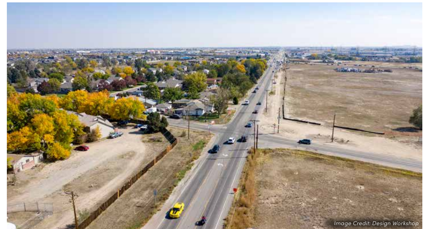
Figure 57: Brighton Road intersecting 104th Avenue
