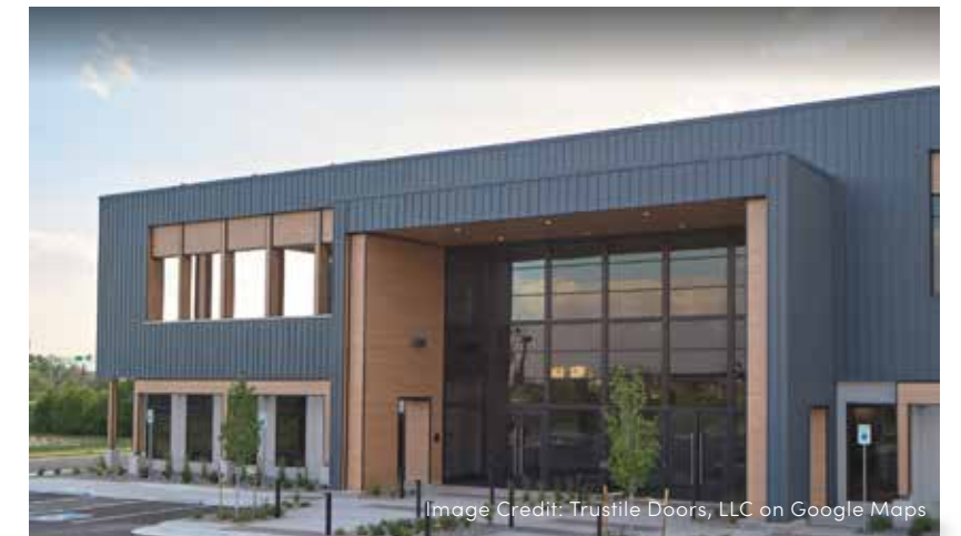
Figure 38: TruStile Doors New Facility
