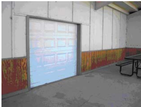
Access to storage below Grandstand
