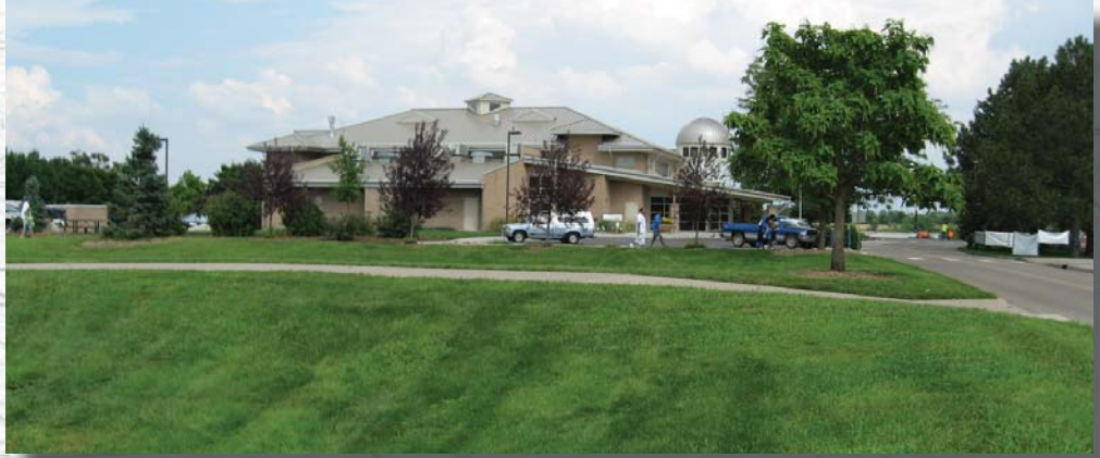
Turf stormwater retention area looking east to Parks Administration building.
