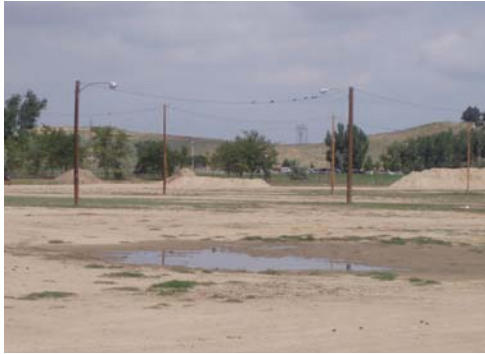
Water ponding in soft surface parking area
