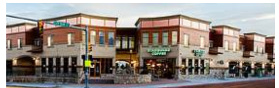
Figure 3: West Park Apartments (Maxiimo Development)
