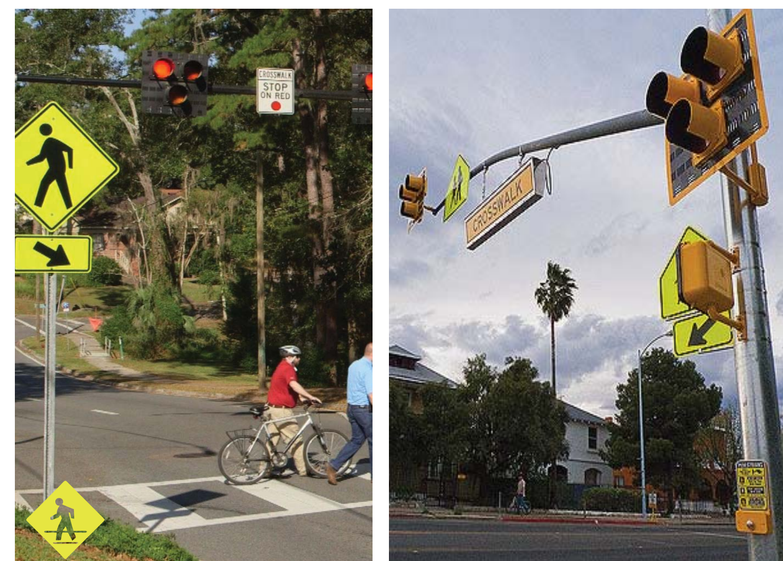
SAFE PLACES TO CROSS - High-Intensity Activated Walk ("HAWK") traffic signals stop traffic when pedestrians need to cross
