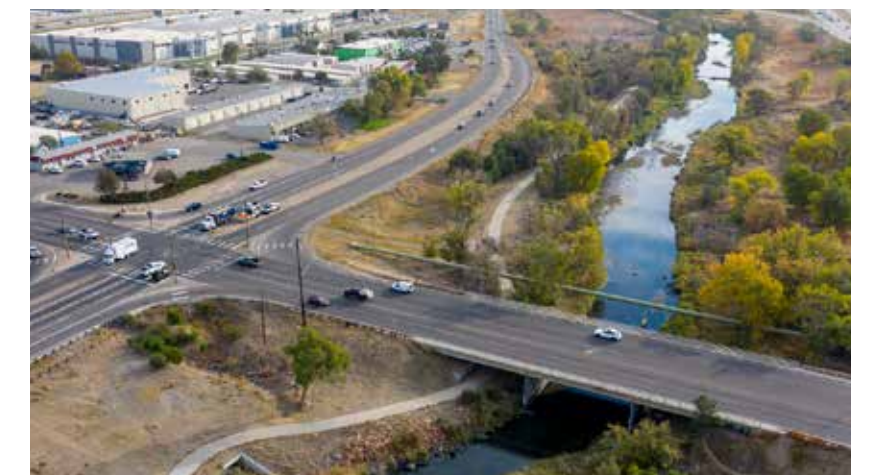
Figure 54: Crossing at Clear Creek Trail
