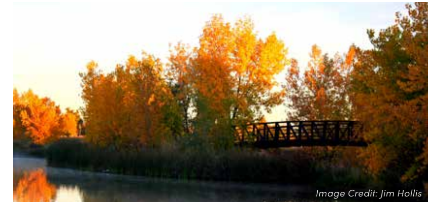
Figure 45: Bridge at Barr Lake
