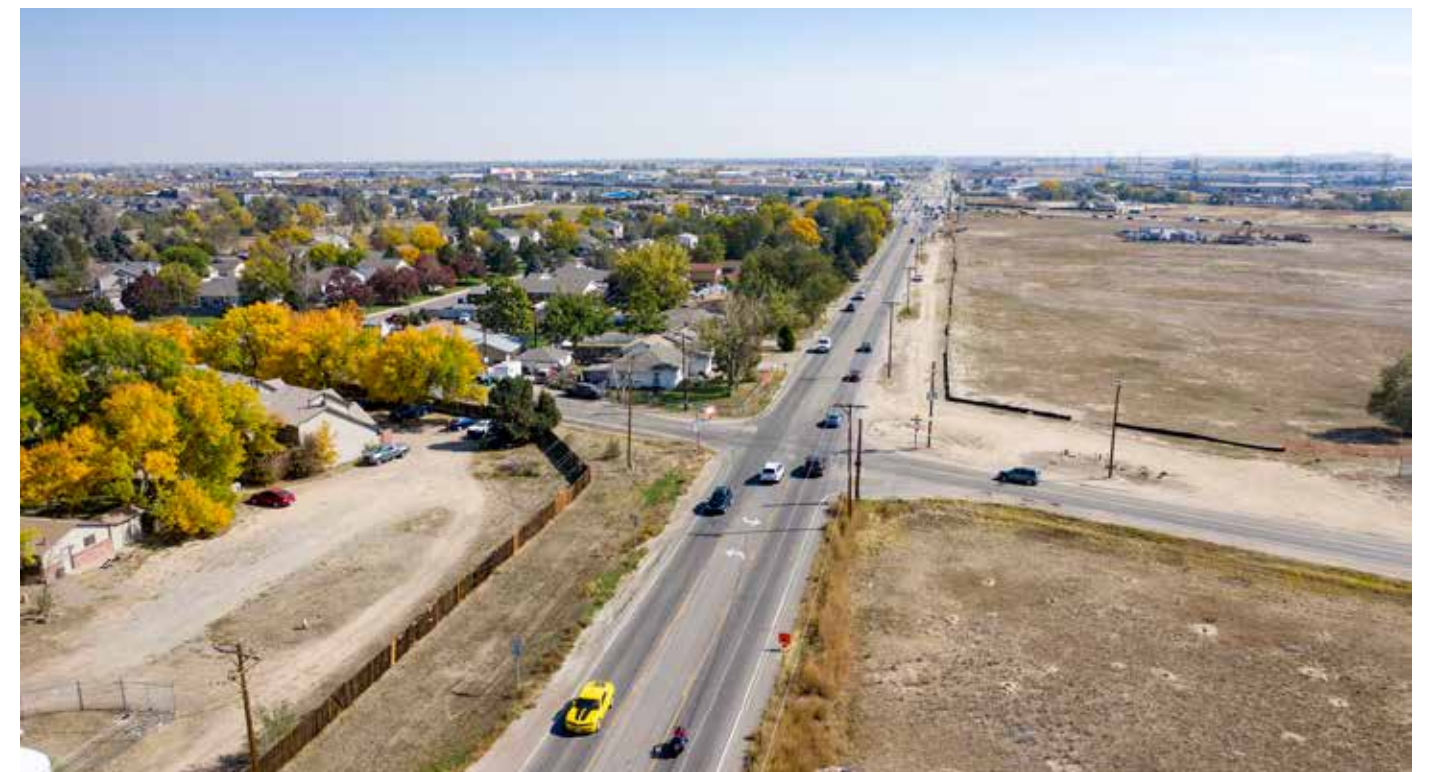
Figure 55: Intersection of Brighton Road and 104th Avenue
