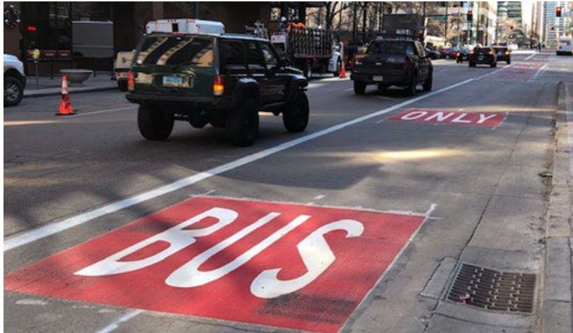
Figure 36: Example of a Dedicated Bus Lane in Downtown Denver (Source: The Denver Channel)
