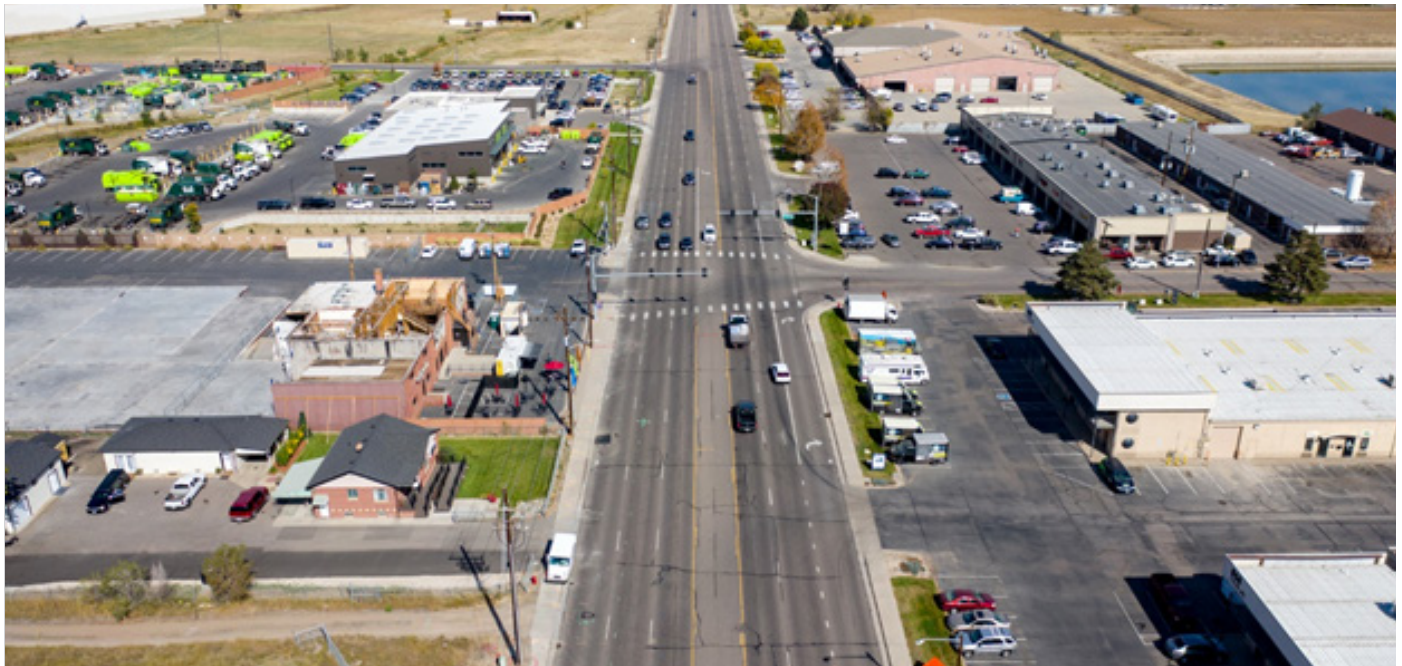
Figure 43: Washington Street Looking North from I-270
