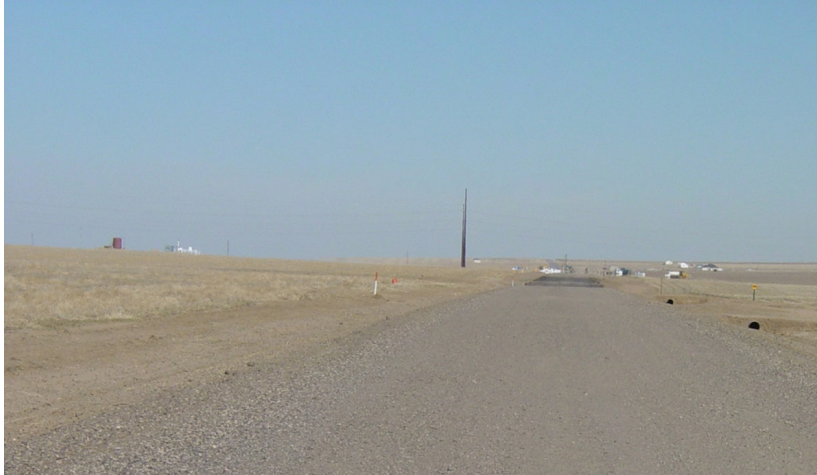
Figure 24: Unpaved Section of Imboden Road
