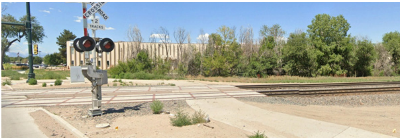
Figure 56: Existing At-Grade Multiuse Trail Crossing on 120th Avenue
