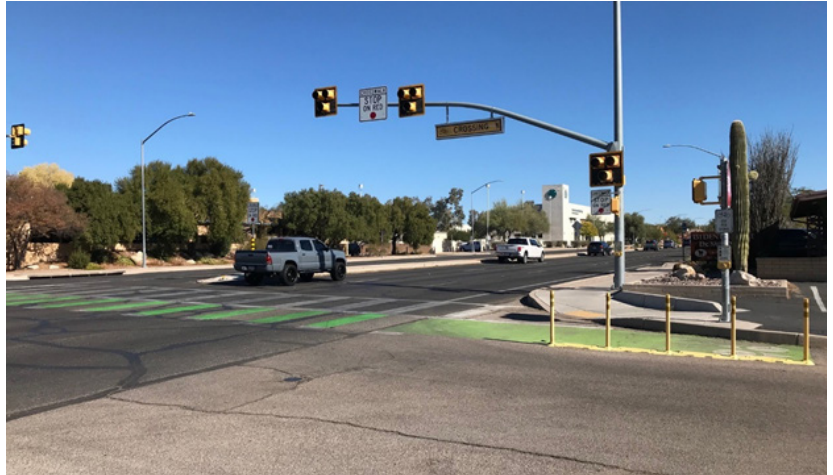
Figure 38: Example of an Enhanced Crossing Treatment with Dedicated Bicycle Striping and Signals
