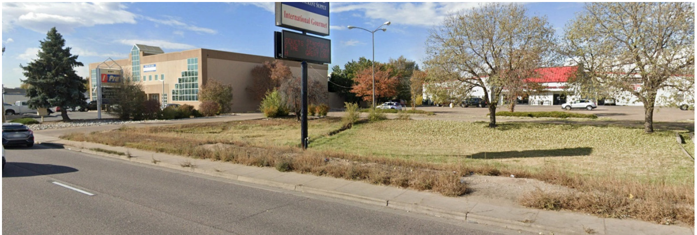
Figure 7: Example of Narrow Sidewalk on Federal Boulevard
