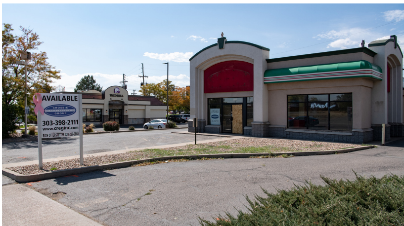
Example of vacant property
